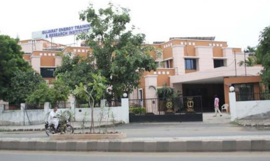
Gujarat Energy Training & Research Institute, Gujarat, Indien
