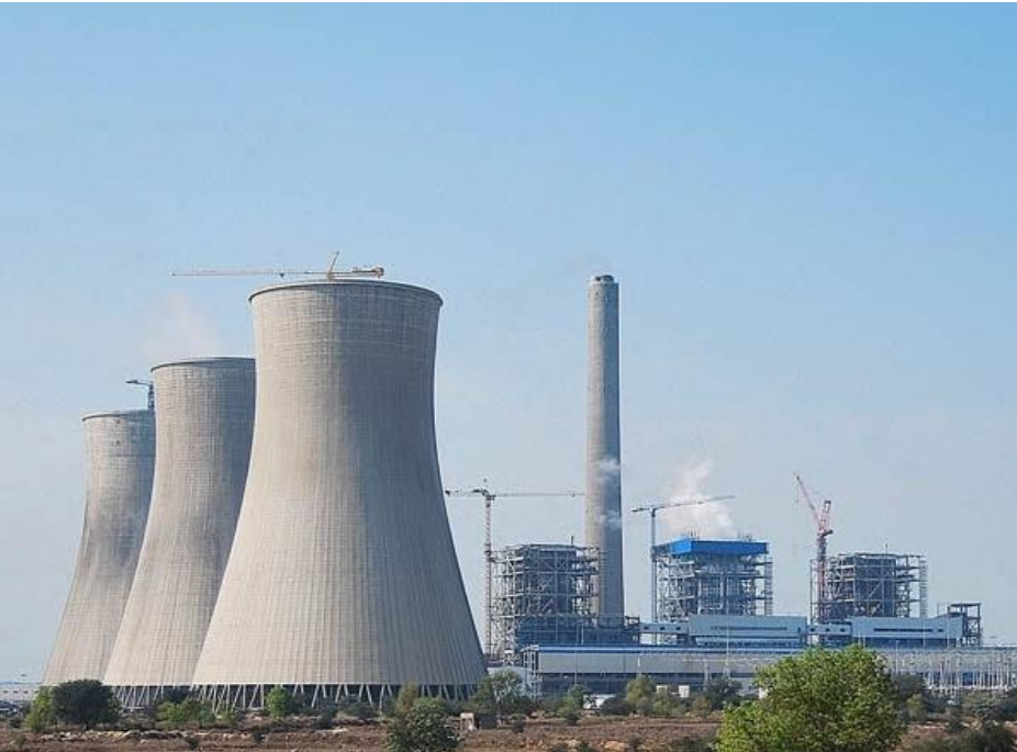
Talwandi Sabo supercritical thermal power plant, Punjab, India
