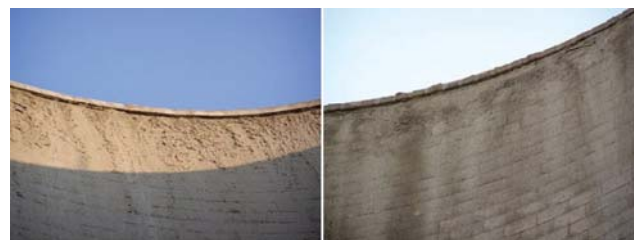
Figure 10. Stack, agglomeration of ash particles.
