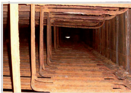
Fig. 2. Unit A: Cleaned supporting tube bulkhead.
